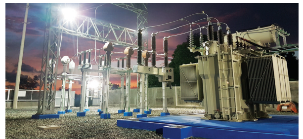
Zambales II Electric Cooperative, Inc. (ZAMECO II) San Marcelino, Zambales 10MVA, 69/13.2 kV Turnkey Substation
