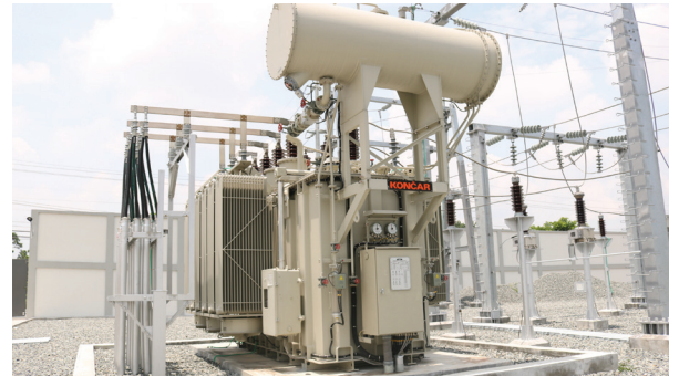
Clark Electric Development Corporation (CEDC) Clark, Pampanga 50 MVA, 69/13.8 kV Power Transformer
