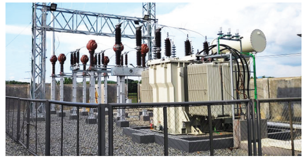
Ilocos Norte Electric Cooperative (INEC) Badoc Substation, Ilocos Norte 10 MVA, 69/13.2 kV Turnkey Substation
