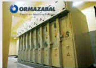
Hermetically sealed and SF6 insulated compact switchgear up to 36kV (Ormazabal, Spain)
