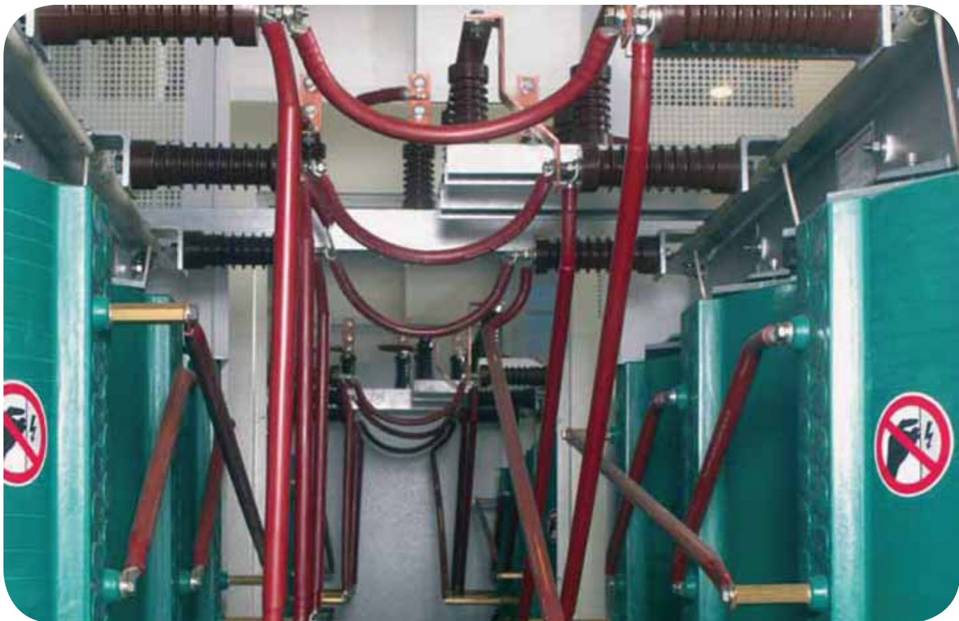
946 kVA 10KV / 2x700V DTR 101000 12 pulse rectifier transformer with phase shift +/- 7,5°
